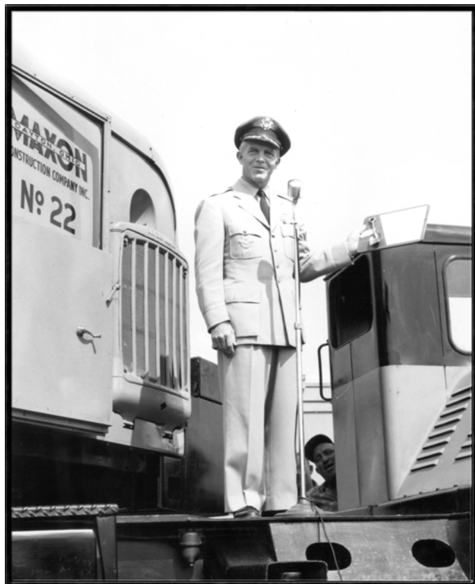
General Watson at groundbreaking in 1956 for new ATIC headquarters, building 828
